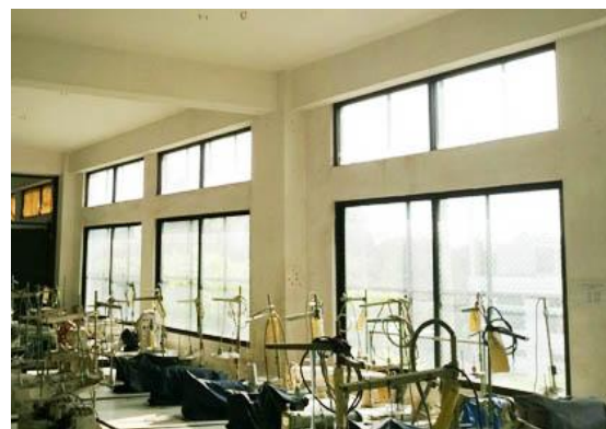
Figure: Sliding window used for ventilation
